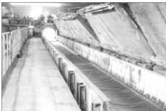
Mubarakheh Steel Complex has a production target of 3.75 million tons in the current Iranian year.
