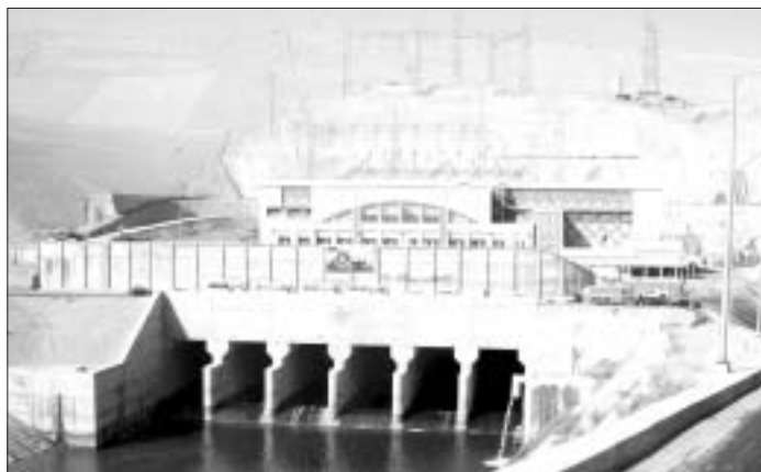
Several hydropower plants are currently in operation, and several more are under construction.
