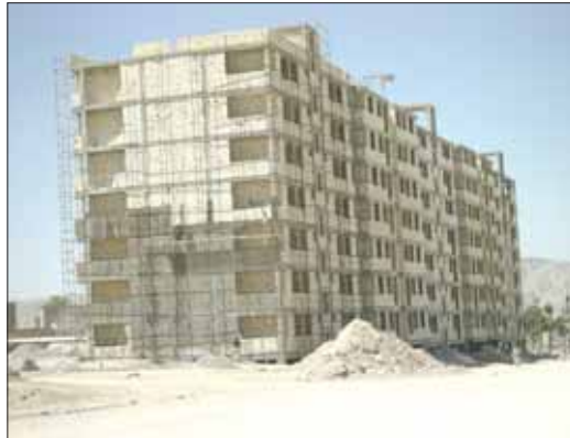
Mass builders should prioritize improving the quality of buildings.
