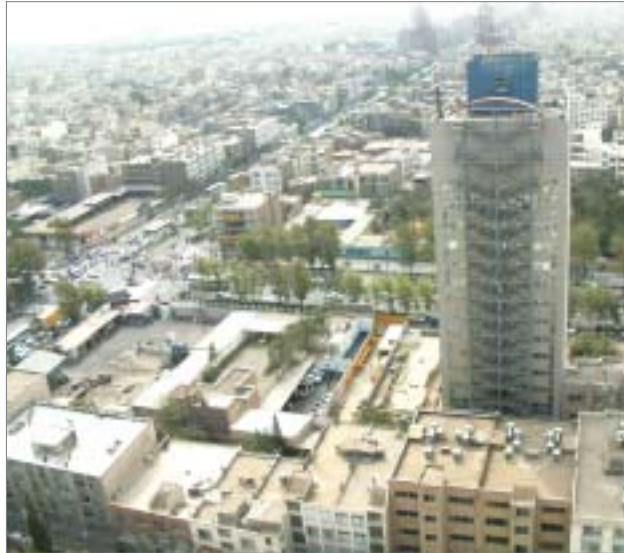
► The regional conference will provide Iran a good opportunity to exchange views with participant delegations on the problems of urban development.
