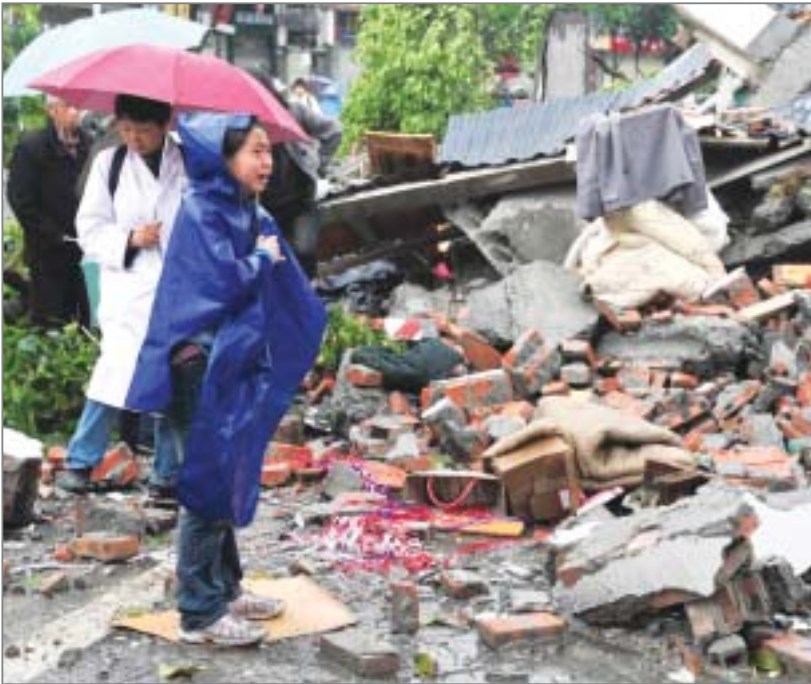
A young Chinese girl weeps in front of a collapsed building in Dujiangyan, May 13.
