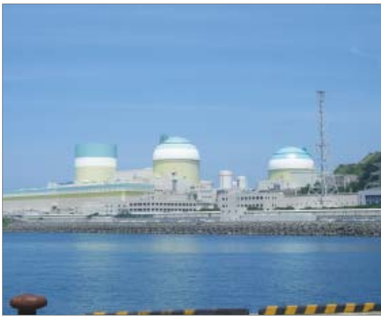
British Energy's eight aging power plants, built since 1965, have been beset by corrosion and other technical problems in the last two years.
